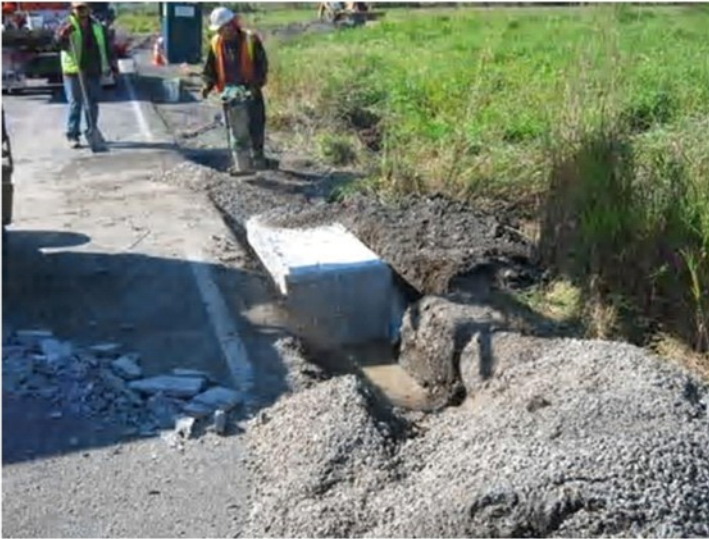
Qwest contractors installing phone cable splice box to reroute Qwest phone cable This took several men and several large machines 3 days work. The work crew had no idea why they were doing it. The City of Enumclaw has to also reroute a water line.
