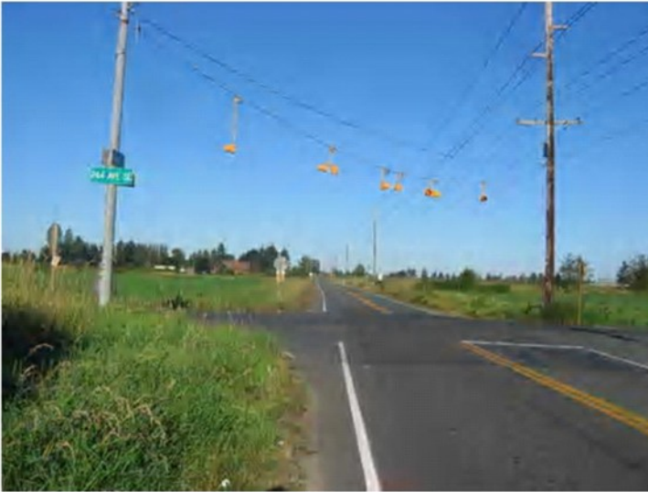
Intersection of SE 416th and 244th SE looking West Before installation of an est. $500,000 concrete fish "roundabout" There are NO problems at this intersection! NO safety problems, NO water problems & NO fish.
